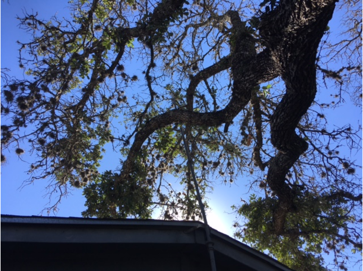
Existing Mobile Home / Tree # 2007 28491 RR-12 / November 28, 2021
