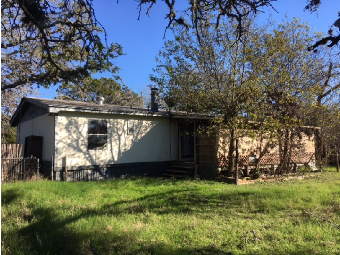
Existing Mobile Home / OFR Frontage / 28491 RR-12 / November 28, 2021
