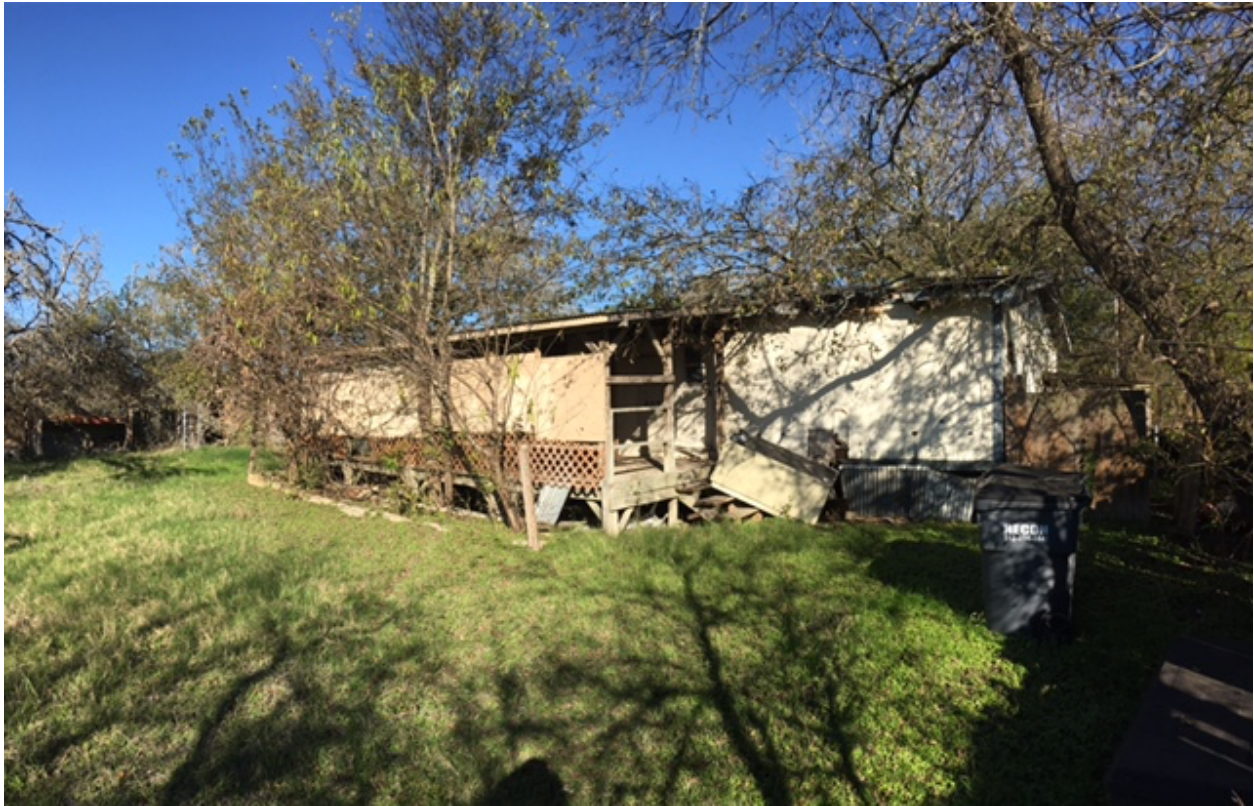
Existing Mobile Home / OFR Frontage / 28491 RR-12 / November 28, 2021
